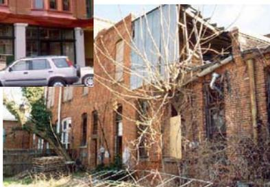
Roof leaks and the collapse of a second story area resulted in extensive damage to the first floor areas. The remainder of the building was generally structurally sound, but the second floor required emergency stabilization to prevent a collapse, and the back wall of the building and the roof structure required stabilization. The City was also concerned that the vacant building would continue to deteriorate and posed a threat to public health and safety. The
